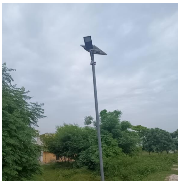
Figure 4: Solar streetlights installed at Khasi Kalan
